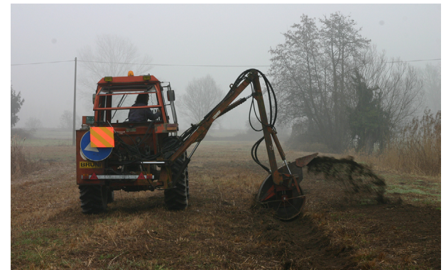
Fig. 61 - Reshaping operations of the ditches - Photo P. Carnaghi
