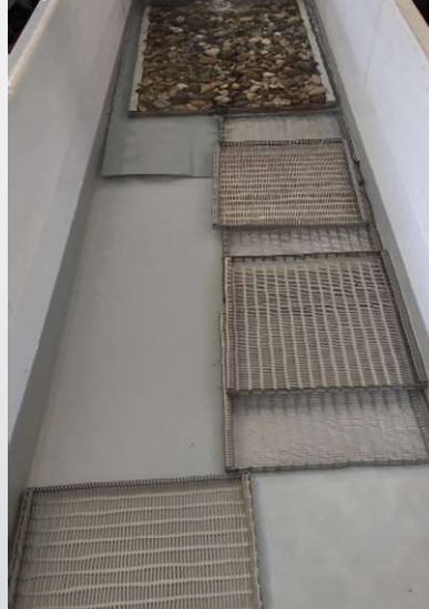
Tanks preparation- Photo by Marco Valenti
