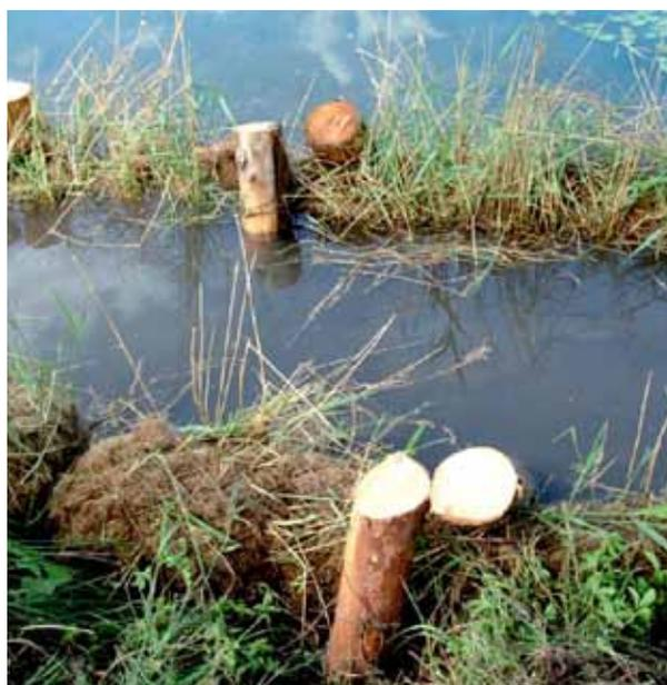
FIG. 6-5 POSA DI RULLI SPONDALI DI CANNETO CON PALI IN CASTAGNO.
